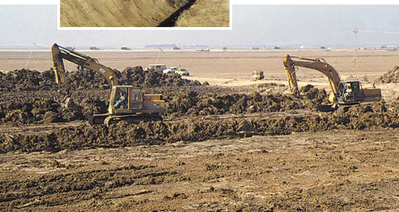
Clean-up of Entremuros area.
