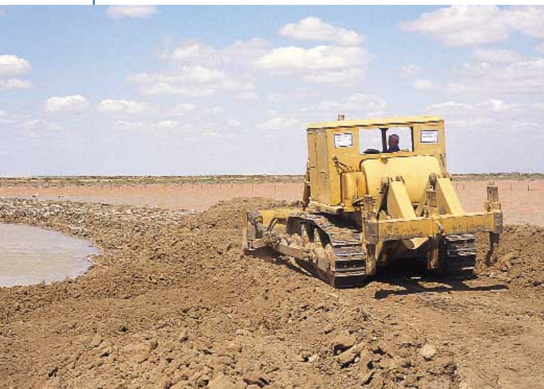
Building of the second dam in Entremuros.
